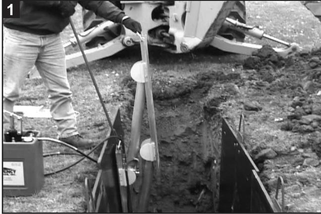
1 Place the shore near the trench edge in the open position with the “cylinder rail” down. Open the valve on the pump can 1/4 turn. Attach the female quick connect fitting on the pump hose to the male fitting on the top cylinder. Put the release tool through the handle on the lower rail with the hook positioned to grab the handle. Fold the shore by pulling the top rail toward you by hand. Lower the shore into the trench with hook.
