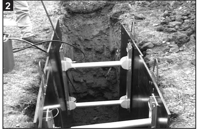
2 Release the top rail and allow shore to completely unfold. The shore will lock itself into open position.
